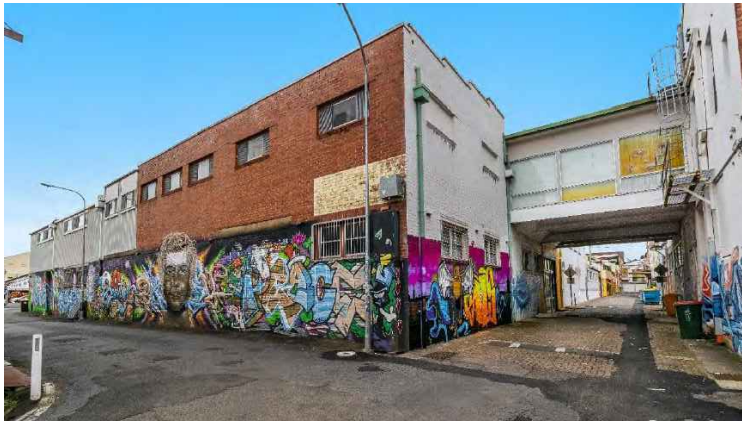
EXISTING BUILDING FROM THE INTERSECTION OF LARKIN LN AND EGGING LN
