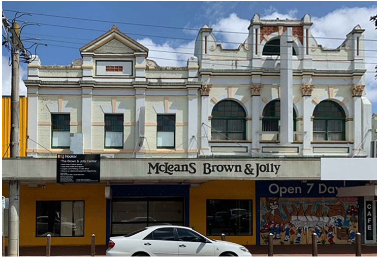
EXISTING BUILDING FROM WOODLARK ST
